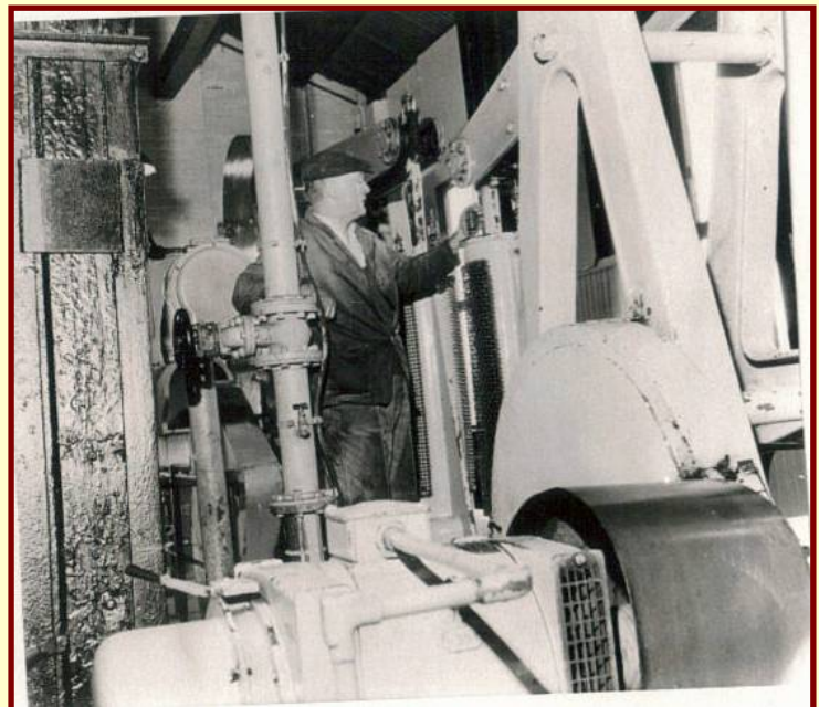
No 1 and 2 pumps operated until 1977, supplying brine to the Elworth Plant
