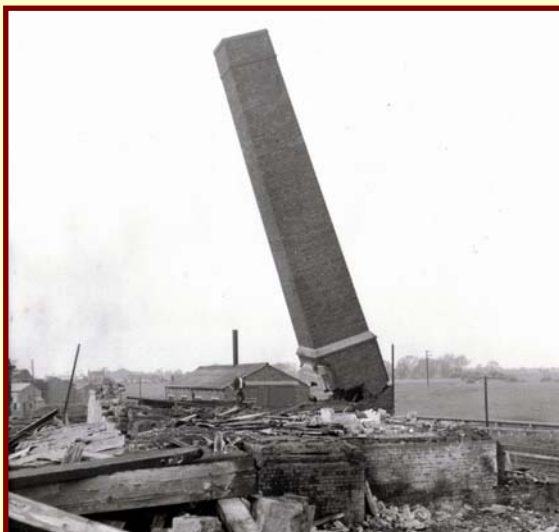
Demolition of no. 8 & 9 Salt Pans Chimney, April 1968
